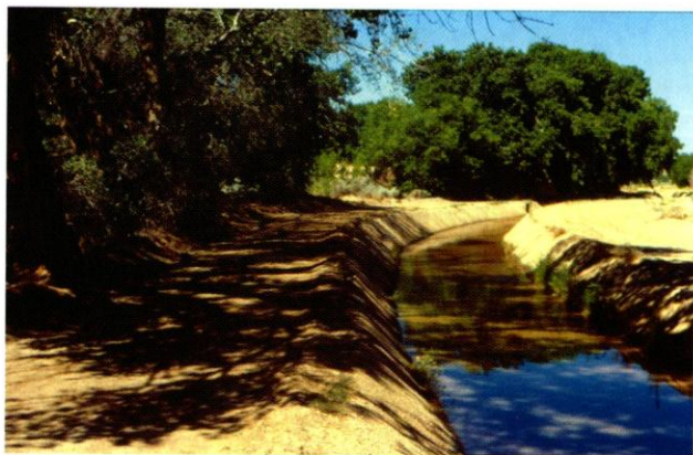
Figure 4 Main Acequia through Corrales.
